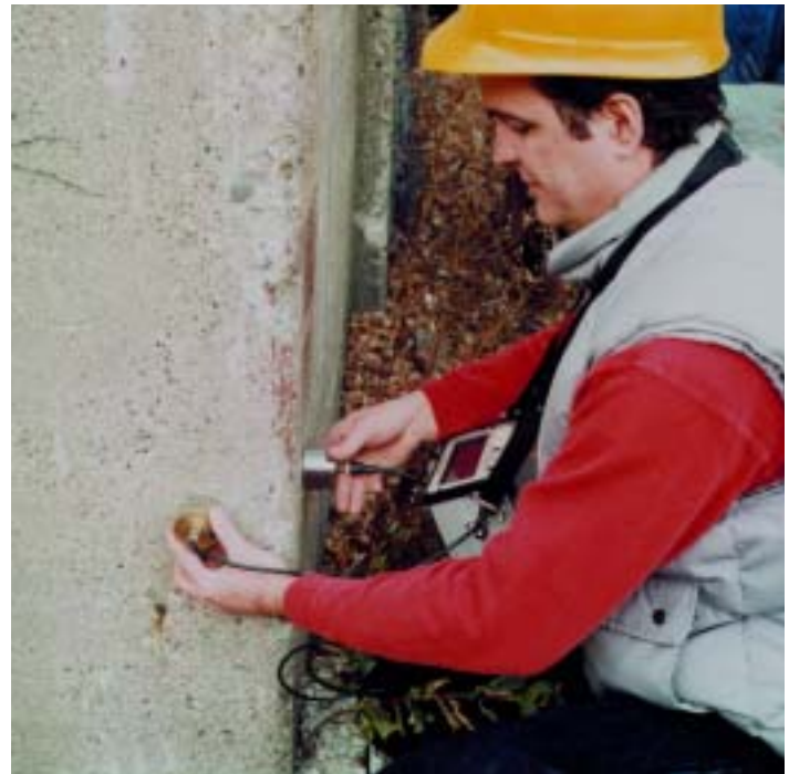
Semi-direct method of checking concrete for flaws.
