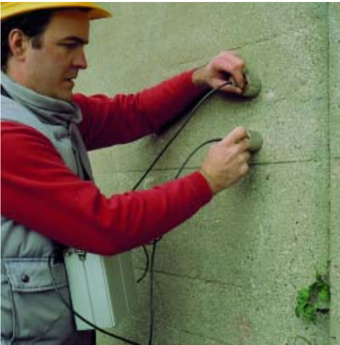
Indirect method: measuring the depth of crack in concrete.
